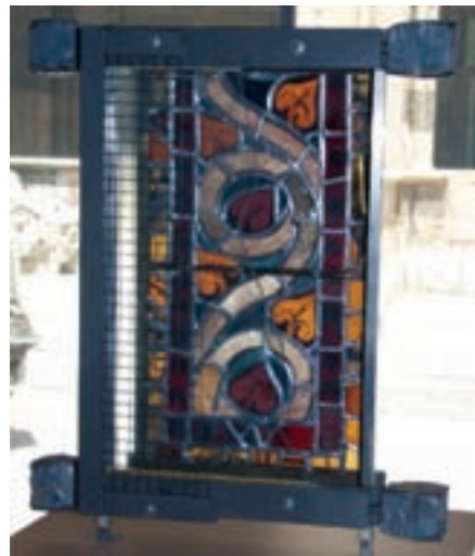
These pictures taken by Andy Lane show how Leon Cathedral puts protective glazing onto its stained glass.
