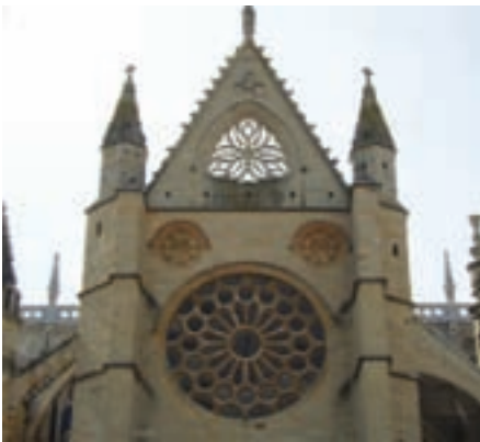
North Gable End of the cathedral.
