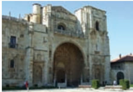
The facade of the chapel of the Parador.
